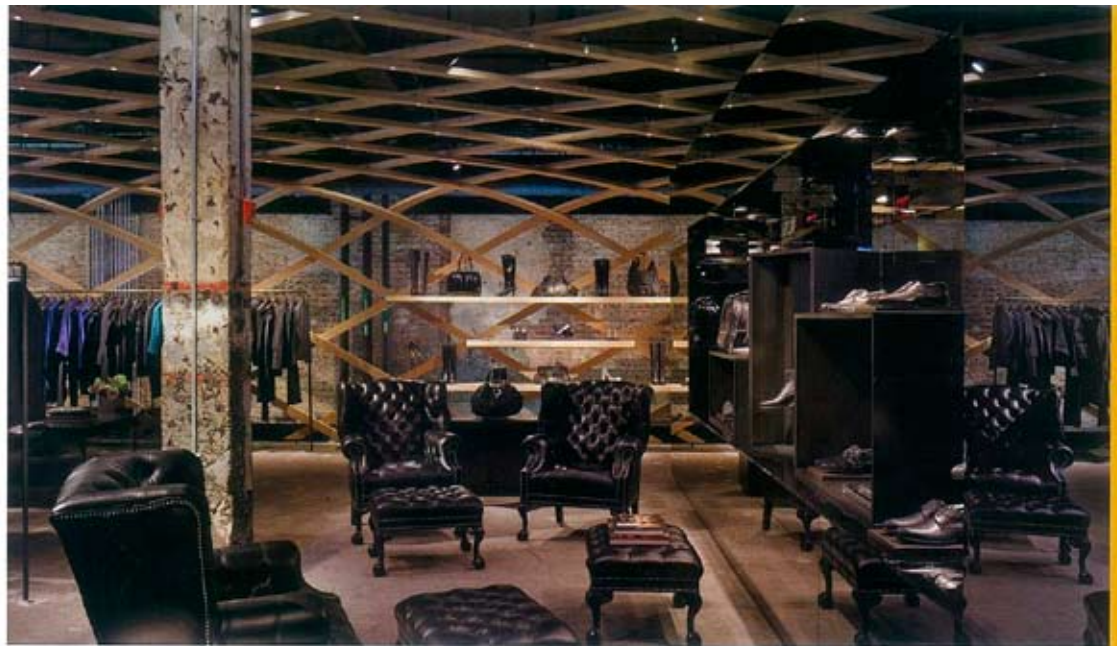
A white LED Kelvin mixing system washes the brick wall and columns, reflected in the focus wall (above). A sequenced system controls LEDs on the new wall and in the lattice ceiling (left).
